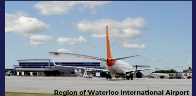
Region of Waterloo International Airport
