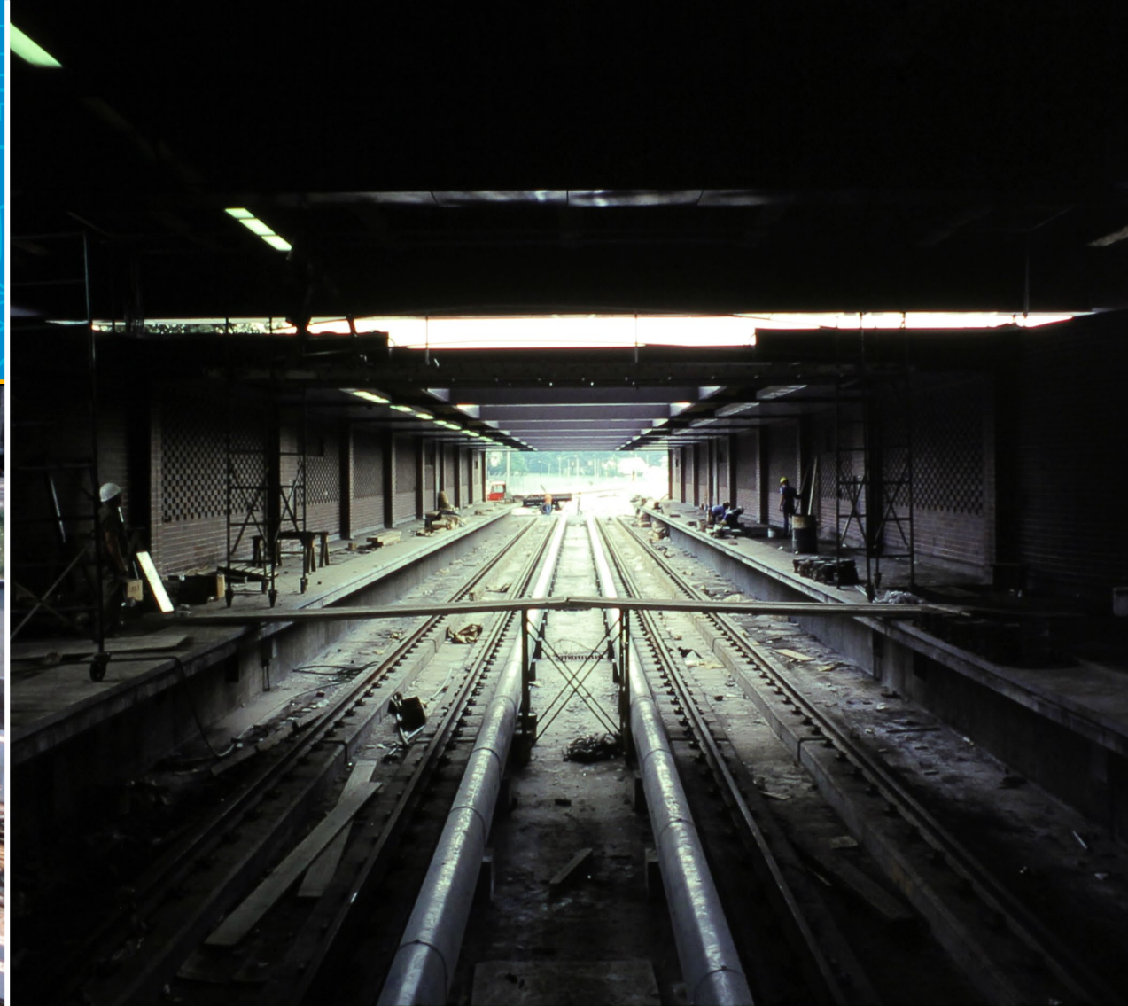
Above: construction of the guideway and platforms at Inman Park/Reynoldstown Station.
