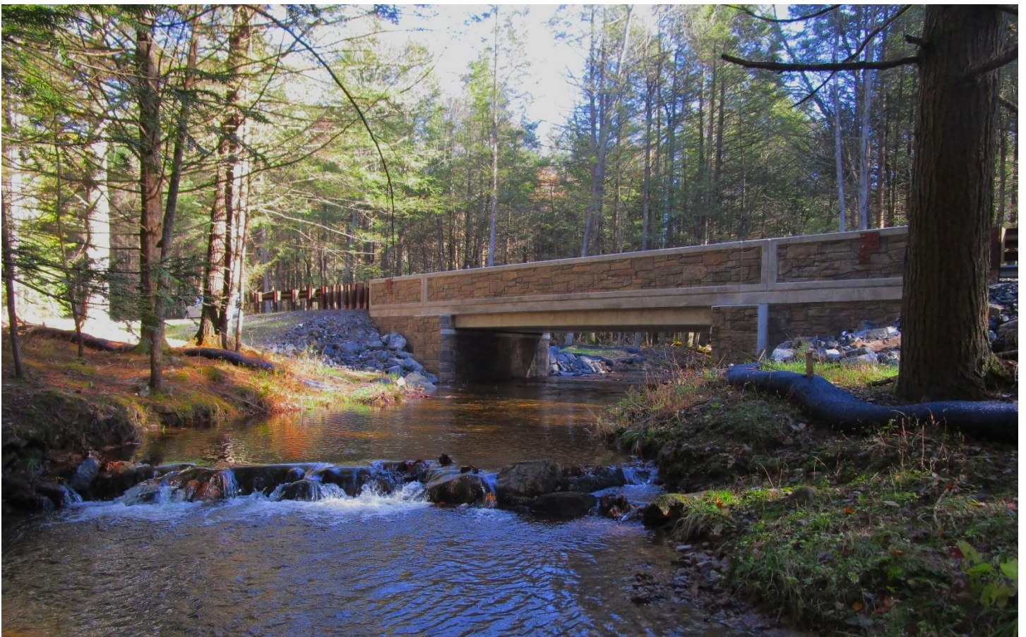
DCNR: Stony Run Road over Pine Creek in Bald Eagle State Forest, Center County, PA
