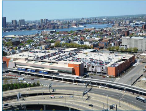
Consolidated Rental Car Facility Logan International Airport East Boston, MA
